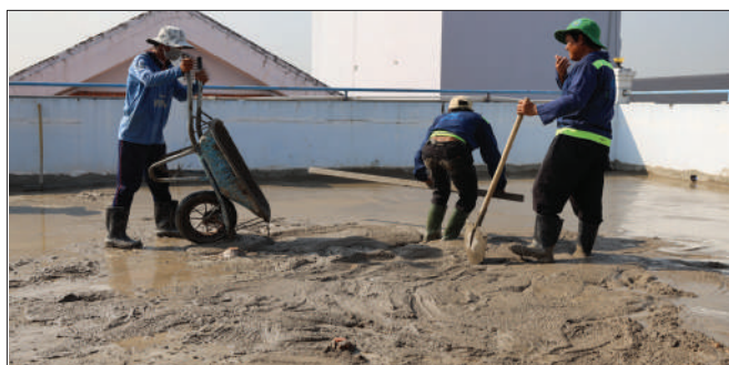
Workers applying concrete on the rooftop
