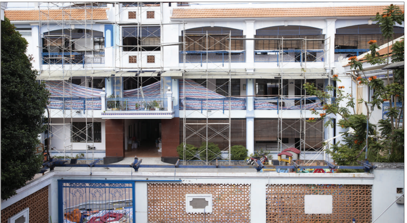
The overview of the renovation at Village Chance
