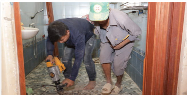
Water-seeping bathroom tiles being removed.
