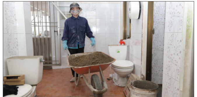
A female worker transferring sand and cement
