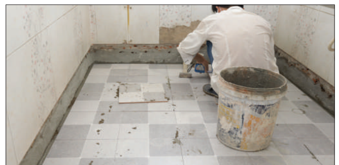
A worker laying tiles in the bathroom
