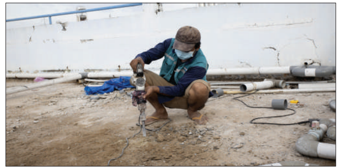
Removing the tiles on the rooftop
