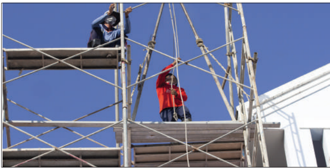
Material is being moved up the roof by the workers.
