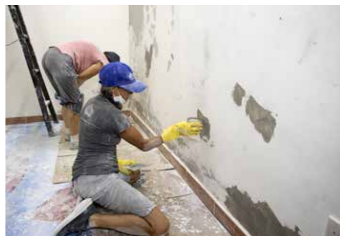
The Casira assists in the renovation of the beneficiary's apartments.
